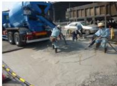
Figure 15. Situation of Casting the Pavement
