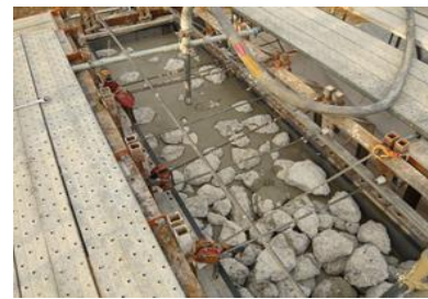
(c) Retaining wall (preplaced-aggregate concrete)
