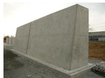
(c) Retaining wall (preplaced-aggregate concrete)
