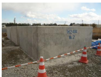
(b) Foot protection block (post-packed concrete)
