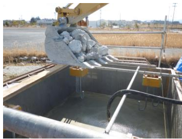
(b) Foot protection block (post-packed concrete)
