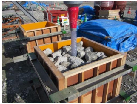
(a) Casting block (pre-placed aggregate concrete)
