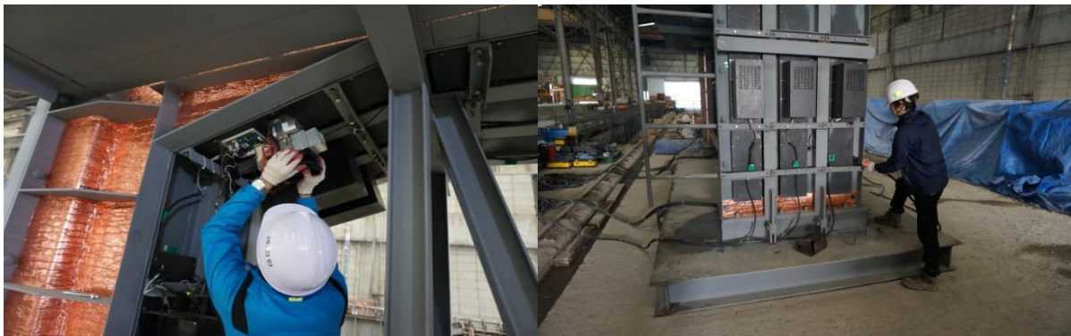
Figure 4. Installation of Microwave Heat Curing Systems to the Form
