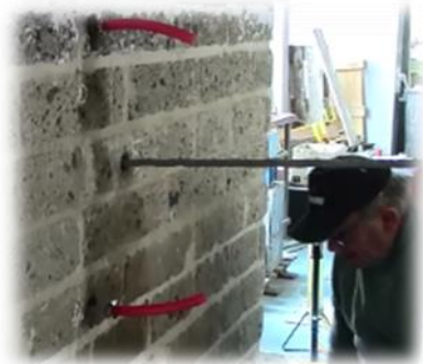
c) Insertion of reinforced CFRP tubes
