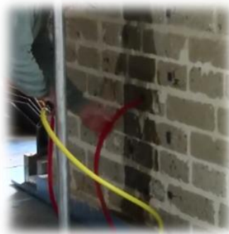
b) Filling of holes
