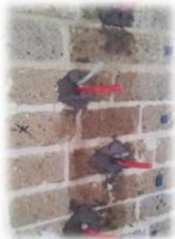
d) Sealing of holes
