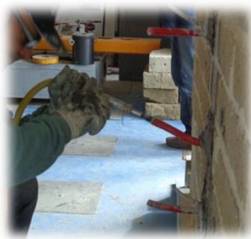
e) Injection of mortar
