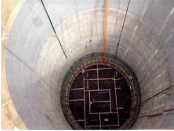
Fig. 1: The foundation slabs for the pumping station were constructed at the bottoms of 70 m (230 ft) deep shafts
