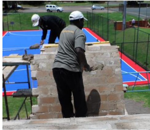
(b) Catenary vault construction
