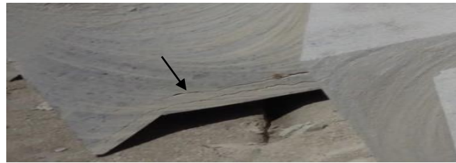
Figure 4. Horizontal cracks
