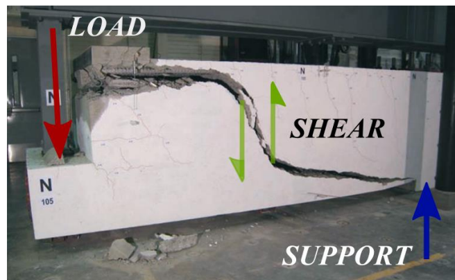
Figure 1. Shear failure in a thick concrete member (Mitchell et al., 2011)
