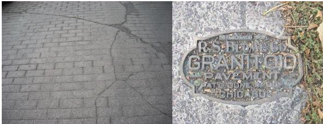
Figure 5. R.S. Blome granitoid pavement in Grand Forks, ND (Hoffbeck, 1990)
