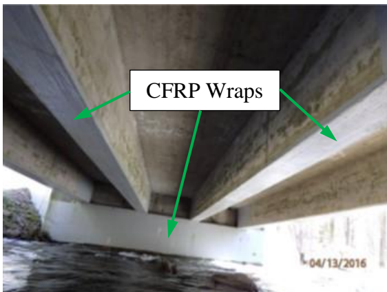
Overview of CFRP wraps in T-beams and an abutment
