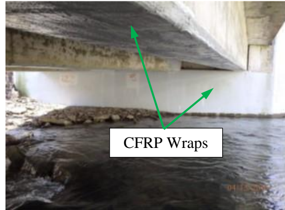
CFRP wraps in abutment #1 and underside of a T-beam
