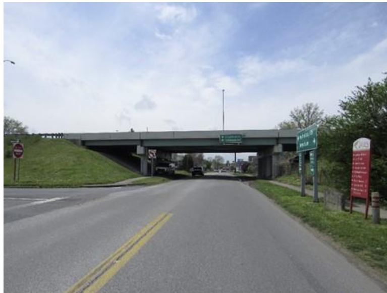
(a) Bridge elevation (looking west) (courtesy: WVDOT 2018 routine inspection report)
