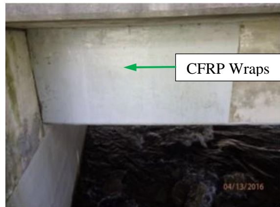
CFRP wraps at the end of a T-beam
