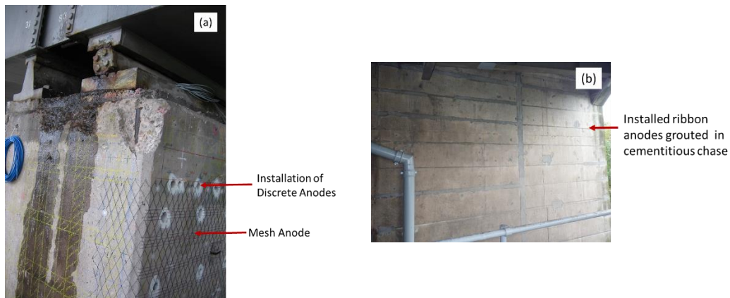
Figure 3: Site images showing anode installation (a) Pier 3 (b) Pier 1 and 2
