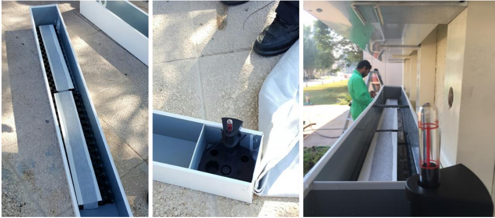
Figure 6: Biofaçades Sub-Irrigation POD System Components Installation (Fadli, F. et al, 2017)
