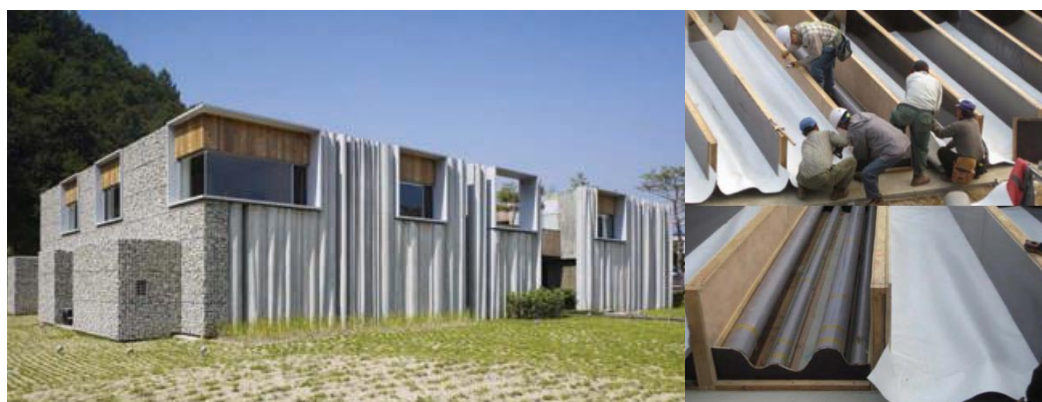
Fig. 1. Fabric formwork construction (Courtesy of Mark West)
