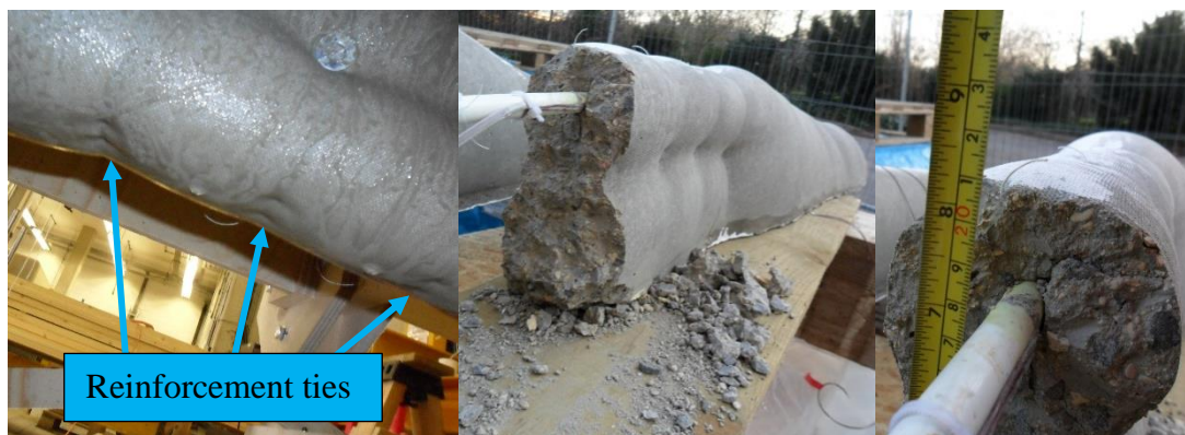
Fig. 8. Glass FRP rebar tied to fabric during construction
