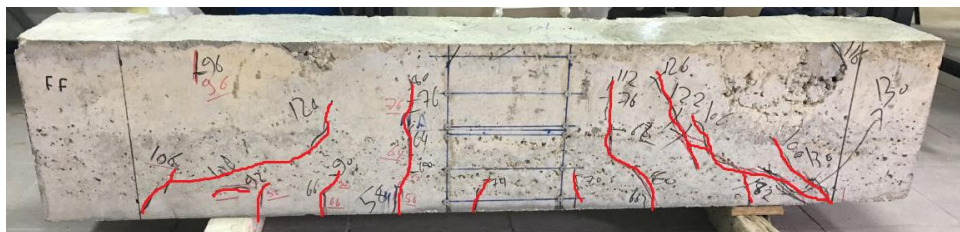
Figure 16. Damage pattern for beam (B3)
