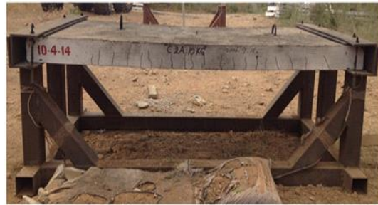
Figure 7. Intact OPSC slab panel after blast with multiple cracks
