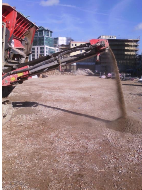
Figure 1: Crushing concrete aggregates on site
