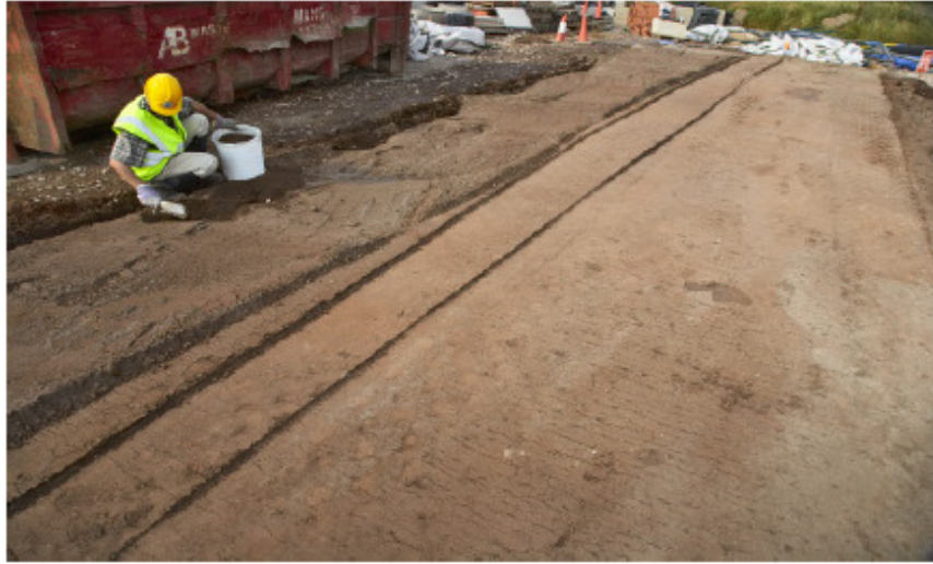
Figure 112. Finished surface of the stabilised soil.
