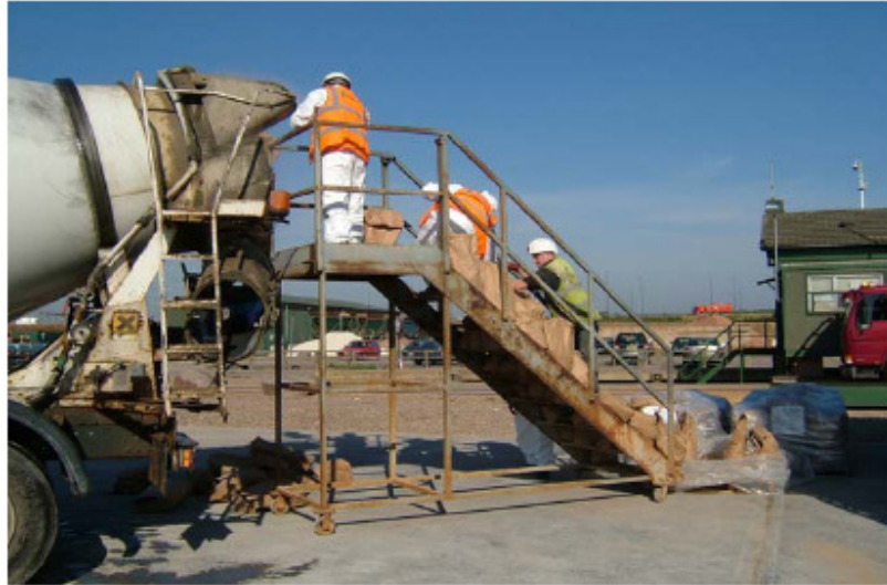
Figure 90. Loading blended binder into the truck mixer.
