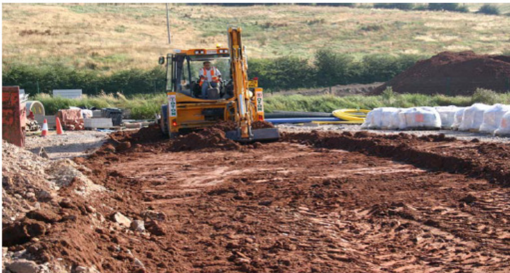
Figure 102. Levelling the spread soil using the JCB.
