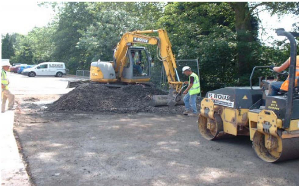
Figure 94. Spreading the concrete using a mechanical excavator.
