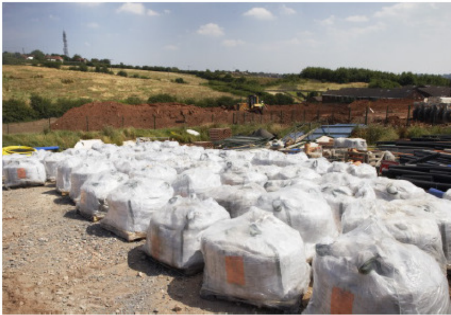
Figure 86. 1000-kg bags of blended powder ready to use (King's Mill Hospital site).
