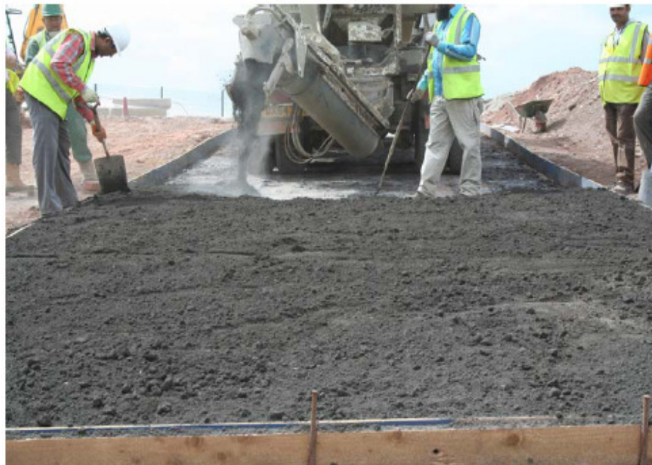
Figure 116. Spreading and levelling the semi-dry paste.
