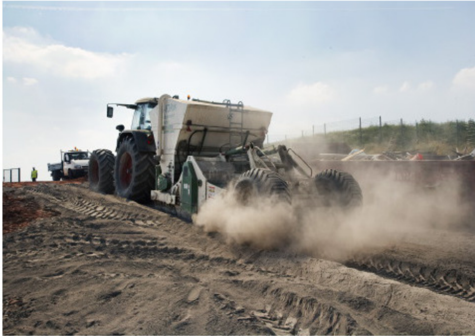
Figure 107. Rotavator in blending position.
