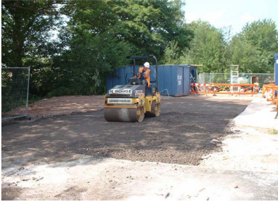
Figure 95. Concrete compaction using a 3-tonne vibrating roller.
