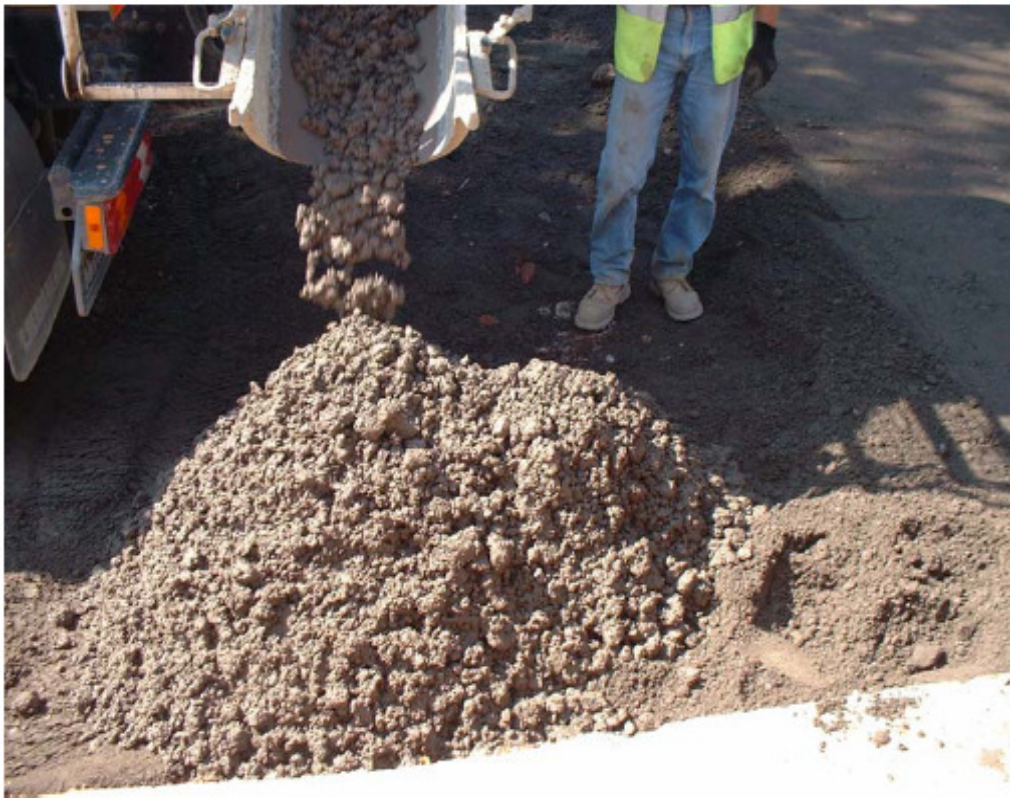
Figure 92. Placing concrete using the truck mixer chute.
