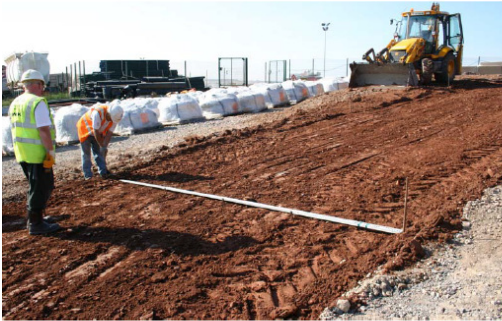
Figure 103. Controlling the accuracy of the thickness of spread soil.
