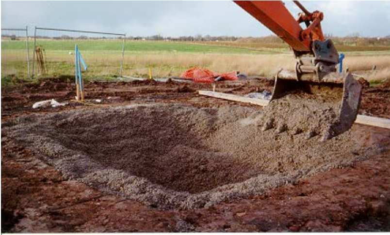
Fig. [7]. Placing concrete in the site trial
