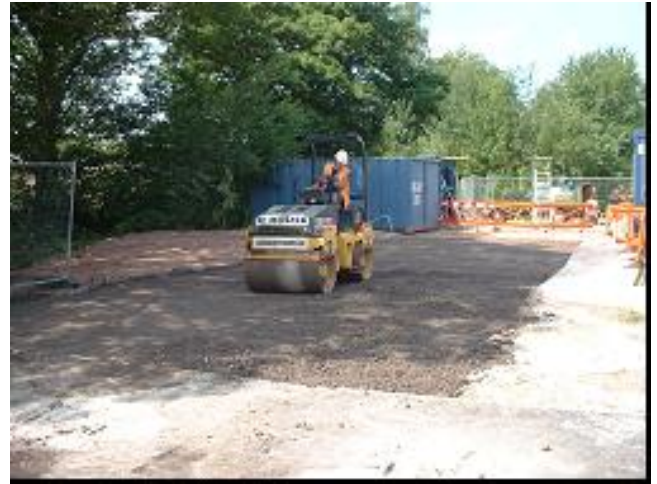
Figure 8. Concrete compaction using a 3-tonne vibrating roller
