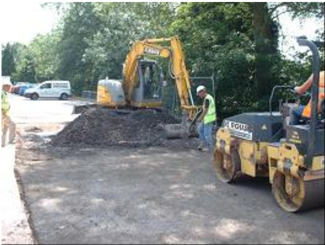
Figure 7. Spreading the concrete using a mechanical excavator
