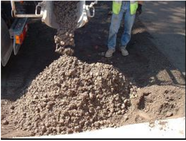
Figure 6. Placing concrete using truck mixer chute
