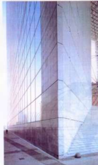
La Grande Arche, Paris. Constructing a 100m cube, 40 storeys high would not have been possible without microsilica technology.
