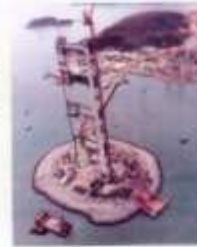
Tung Ma Bridge, Hong Kong. 200m high towers slipformed with microsilica concrete – specified for ease of placement and resistance to an aggressive marine environment.
