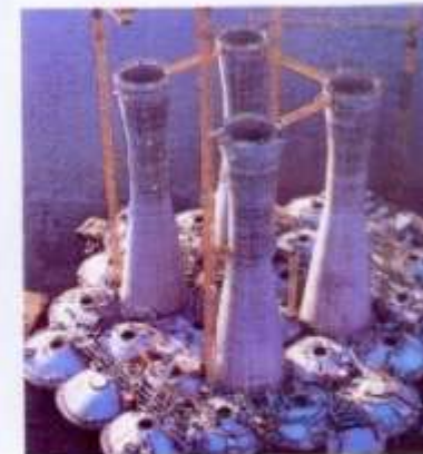
Gullaks C 00 Platform. The innovative construction methods used to build North Sea oil platforms developed around the beneficial pumping properties of microsilica concrete.
