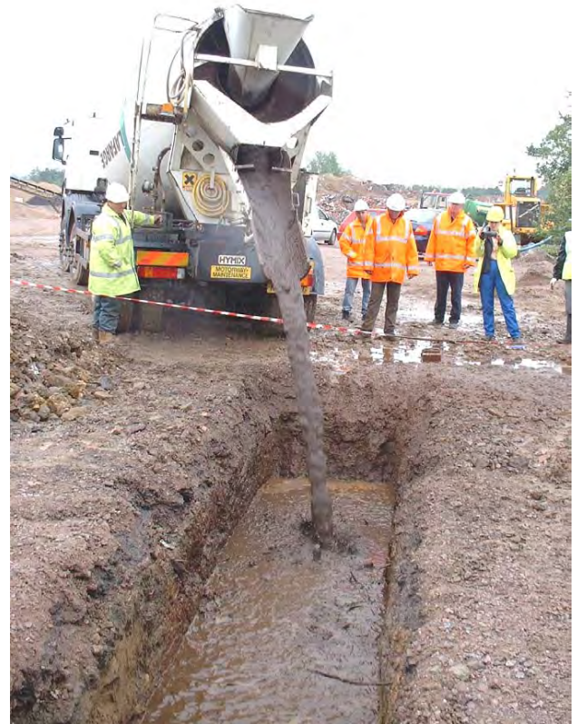
Fig. (19). CLSM Discharge to trench.
