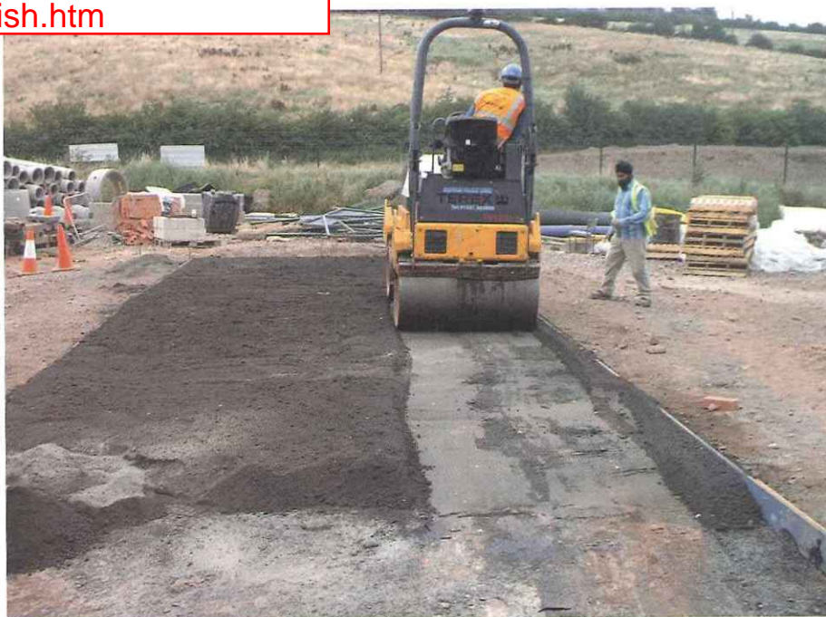
Figure 1: CEM 0 trial with a concrete without aggregate. This semi-dry paste was laid in a 100mm layer.
