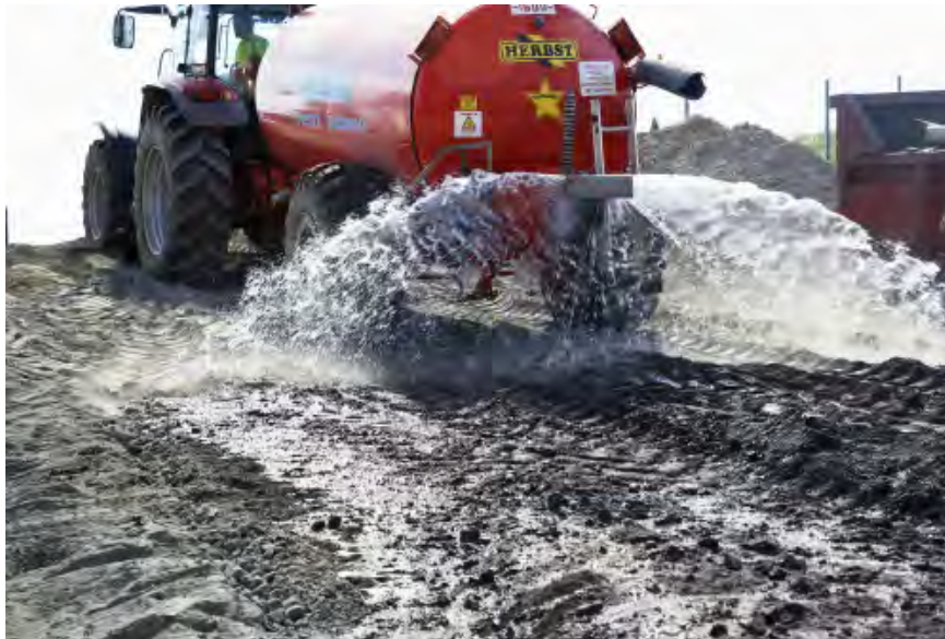
Figure 115 Watering the mixture of soil and the binder using the sprinkler
