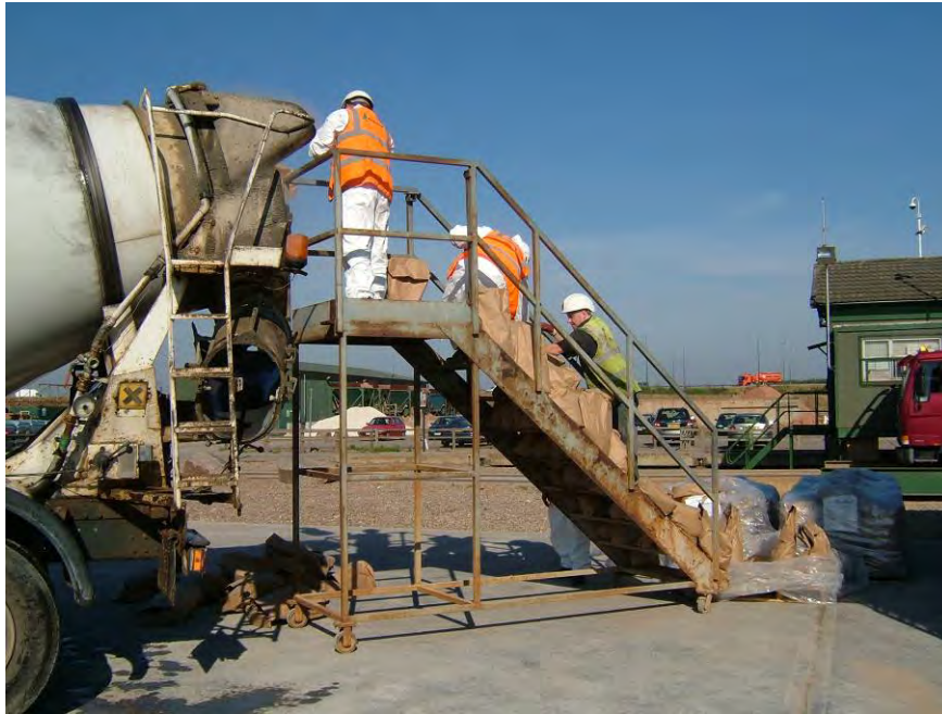
Figure 96 Loading blended binder into the truck mixer
