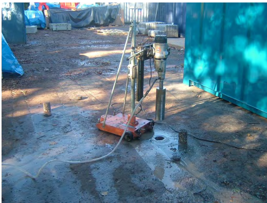
Figure 134 Core sample taken from middle and end part of the trial car park at the Lowdham Grange site
