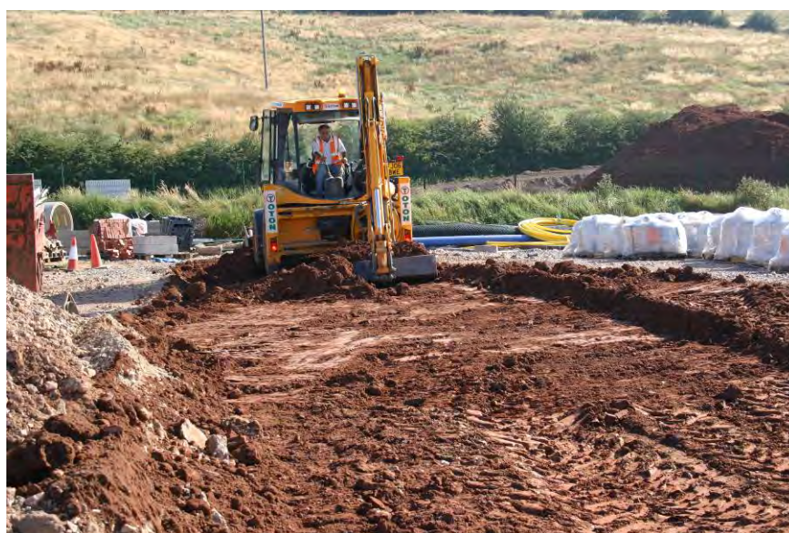
Figure 108 Levelling the spread soil using the JCB
