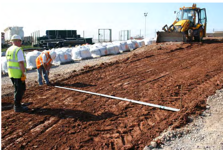
Figure 109 Controlling the accuracy of the thickness of spread soil
