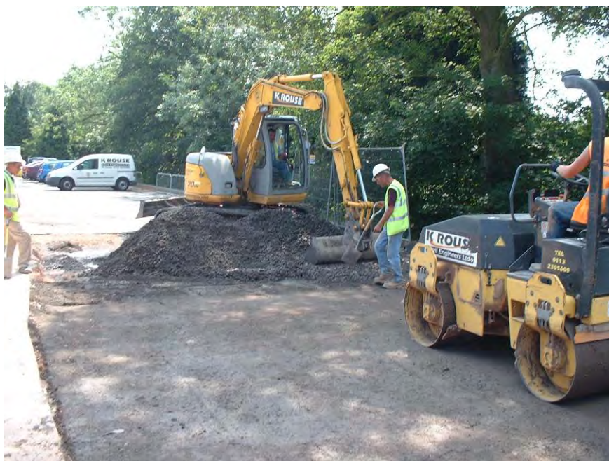
Figure 100 Spreading the concrete using a mechanical excavator
