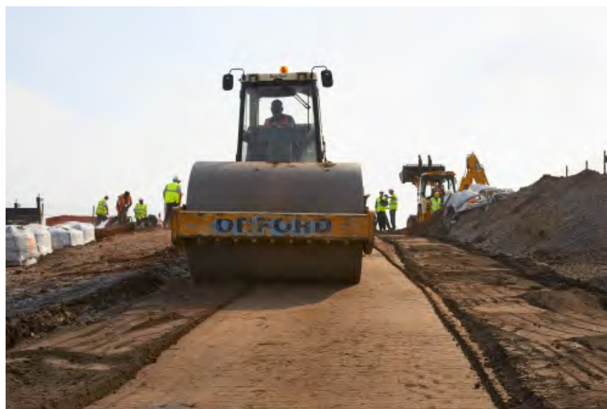
Figure 117 Compacting the blended soil and the binder using the 10-tonne roller
