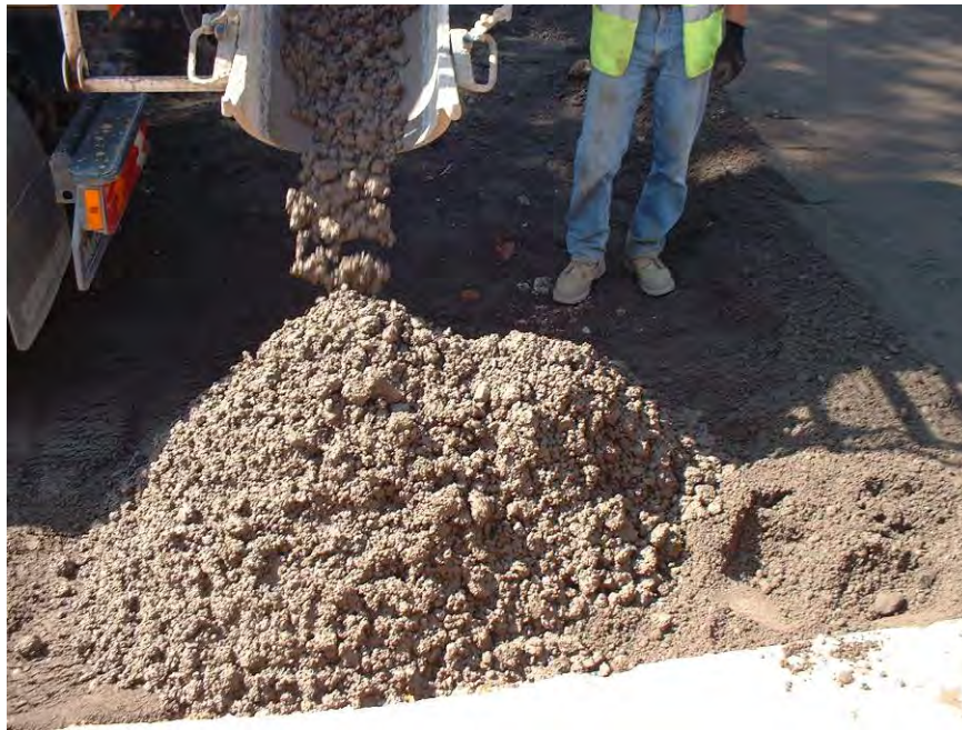
Figure 99 Placing and spreading the last batch of concrete
