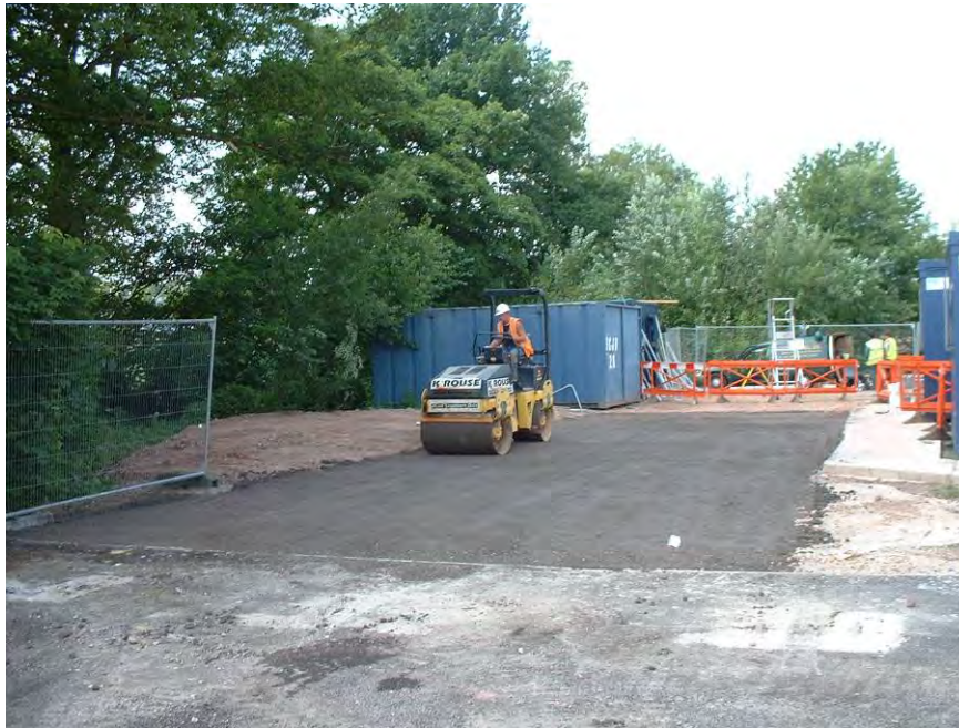
Figure 102 Completed 100-mm layer of RCC at the Lowdham Grange site
