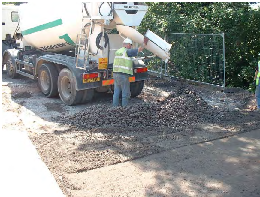
Figure 99 Placing and spreading the last batch of concrete
