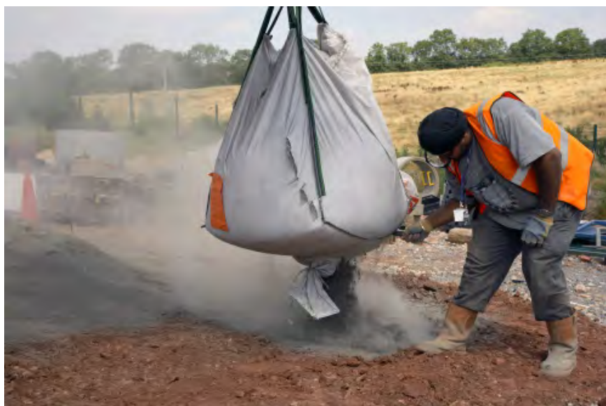
Figure 110 Placing and spreading the powder on top of levelled soil
