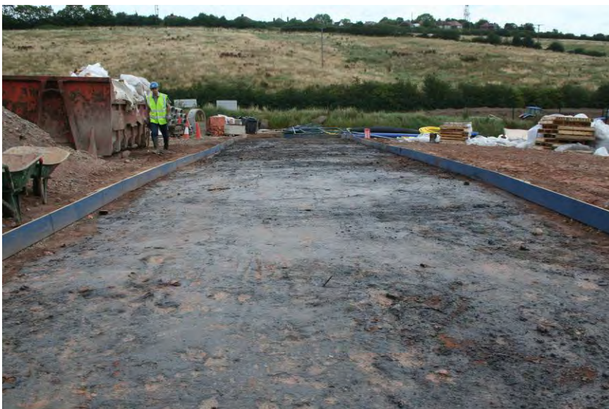
Figure 120 Sprayed surface of stabilised soil before constructing the paste layer
