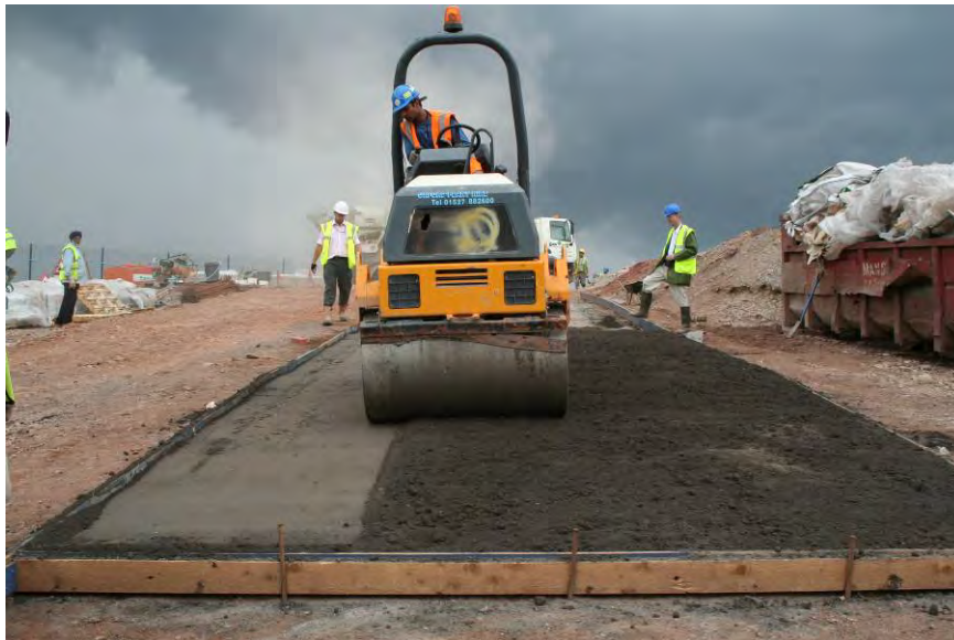
Figure 123 Compacting the semi-dry paste layer using a 3-tonne roller
