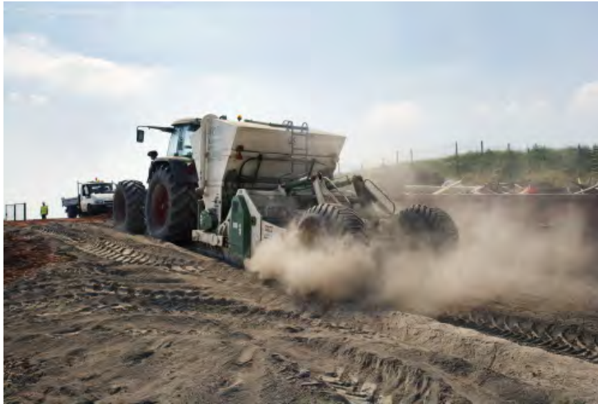
Figure 114 Inspecting the blended soil and powder before adding extra water
