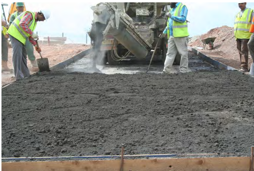
Figure 122 Spreading and levelling the semi-dry paste
