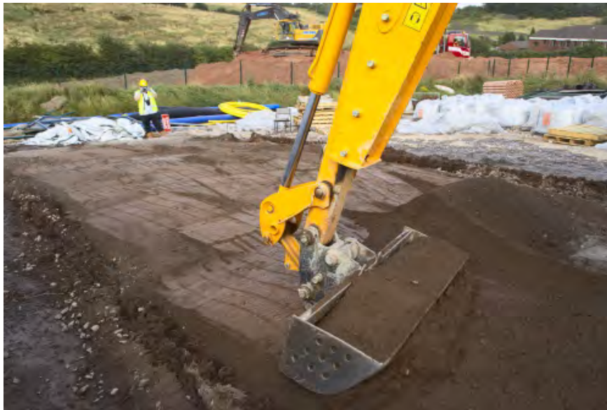
Figure 116 Levelled blended soil and powder ready for compaction
