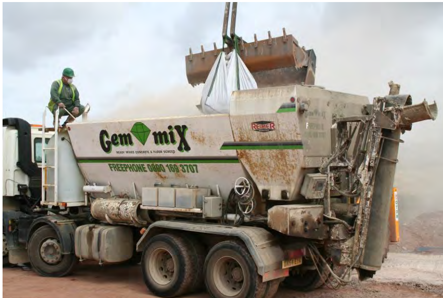
Figure 121 Loading the mixer with blended powder
