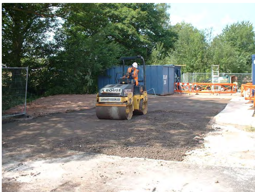
Figure 101 Concrete compaction using a 3-tonne vibrating roller
