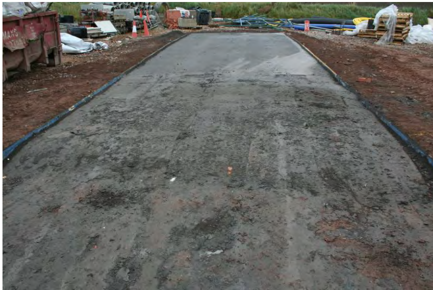
Figure 124 Finished surface of the compacted semi-dry paste
