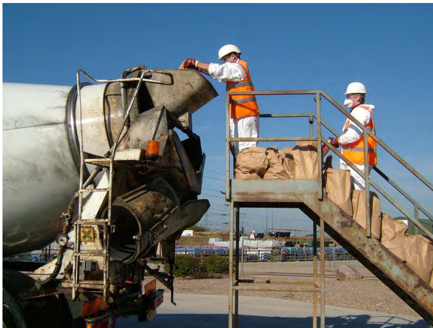
Figure 97 Loading blended binder bags into the truck mixer
