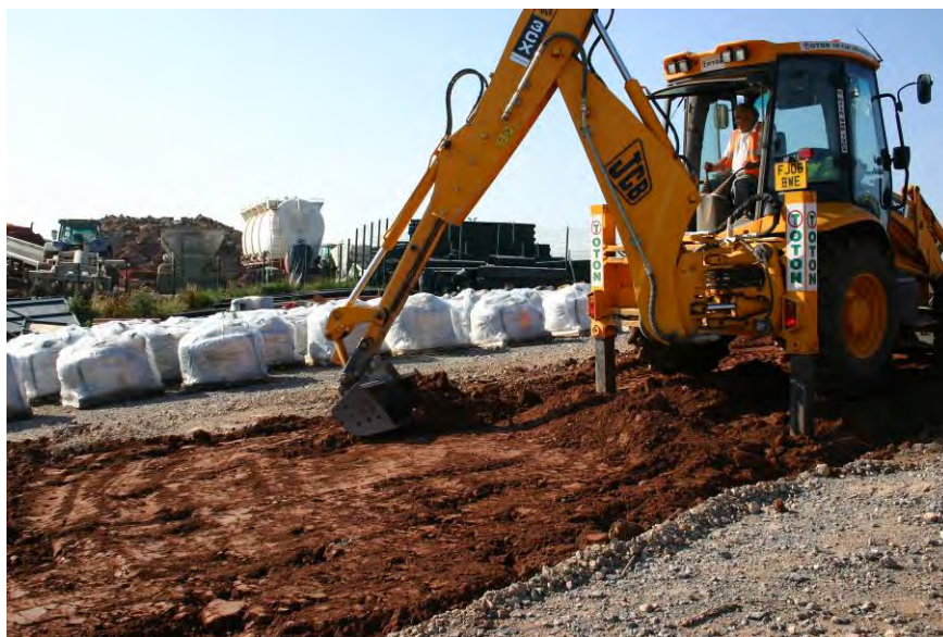
Figure 107 Spreading and levelling the soil in the trial area
