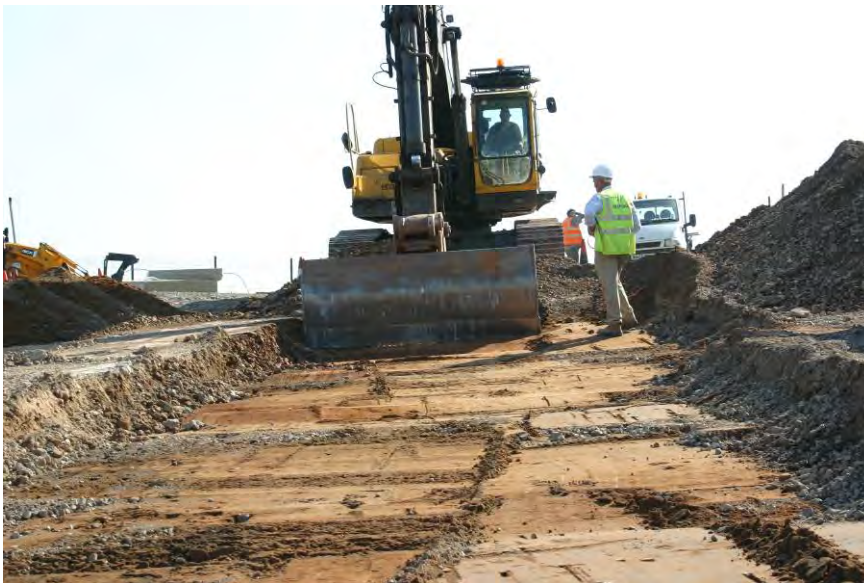
Figure 106 Trimming and levelling the trial area to expose the sub-grade
