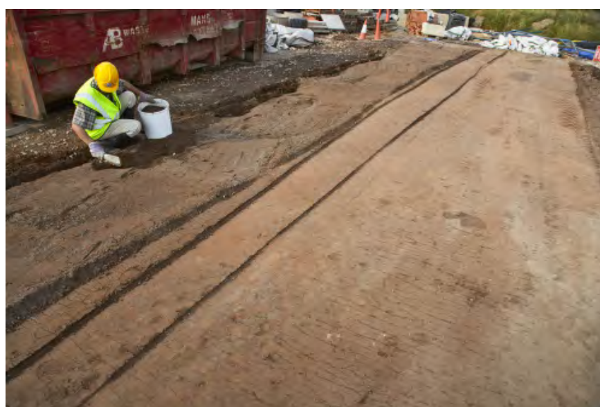
Figure 118 Finished surface of the stabilised soil
