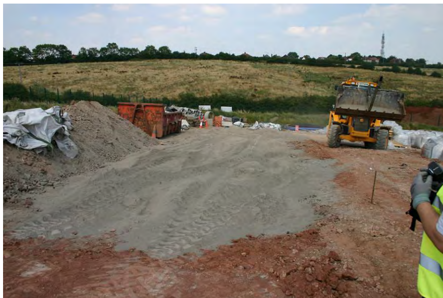
Figure 111 Levelled layer of powder on top of the soil
