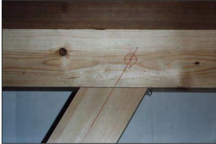
*Figure 4.39 Neutral axes and bolt position are drawn on the timber surfaces.*
