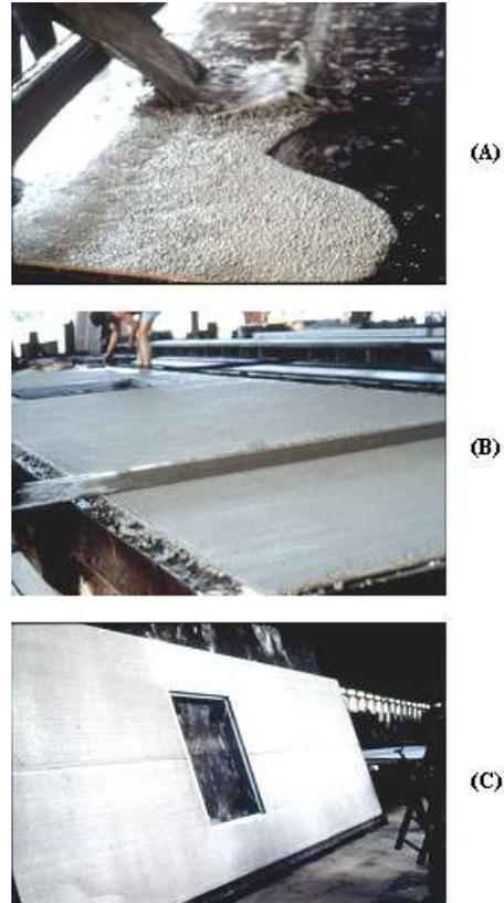
Figure 10. Precast lightweight concrete: casting of SCC (A); Screeding without vibration (B); demolding of the hardened lightweight panel (C).
